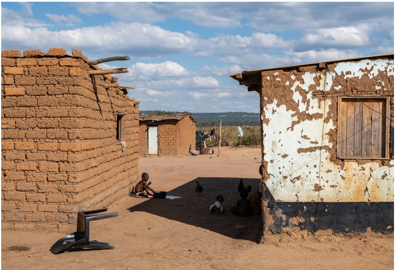
Brick walls and corrugated metal roofs: living conditions are difficult in the villages around the MUMI concession.
